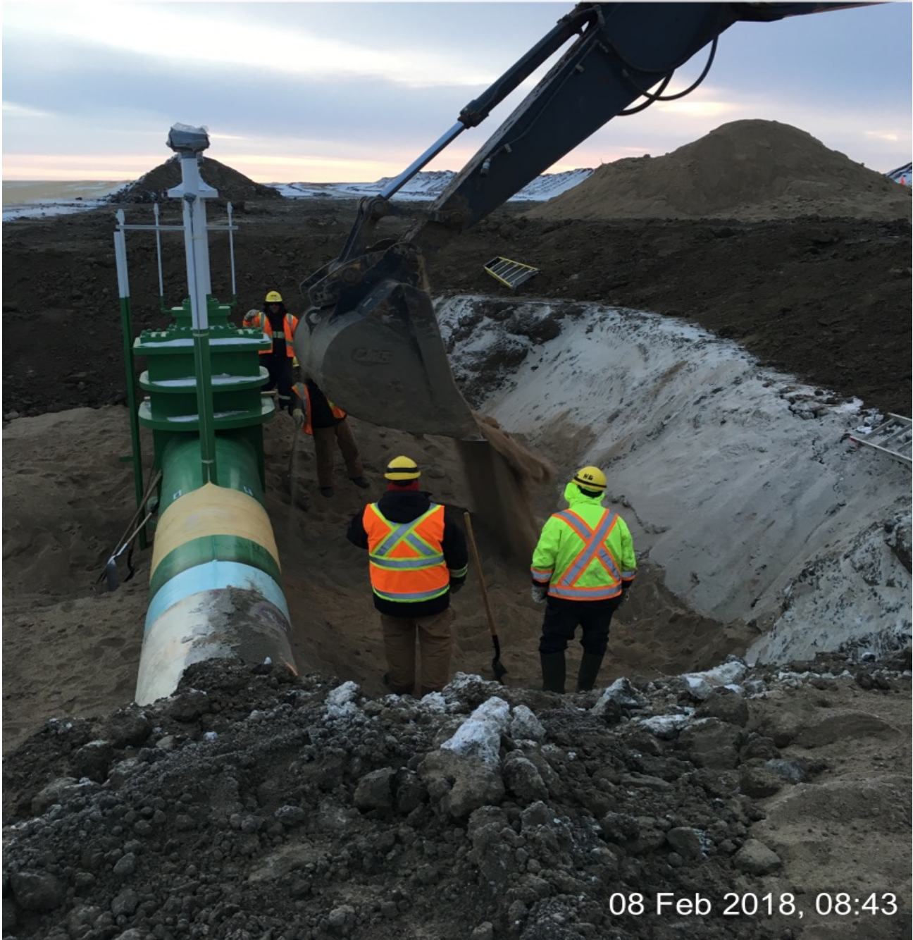
BACKFILLING VALVE
