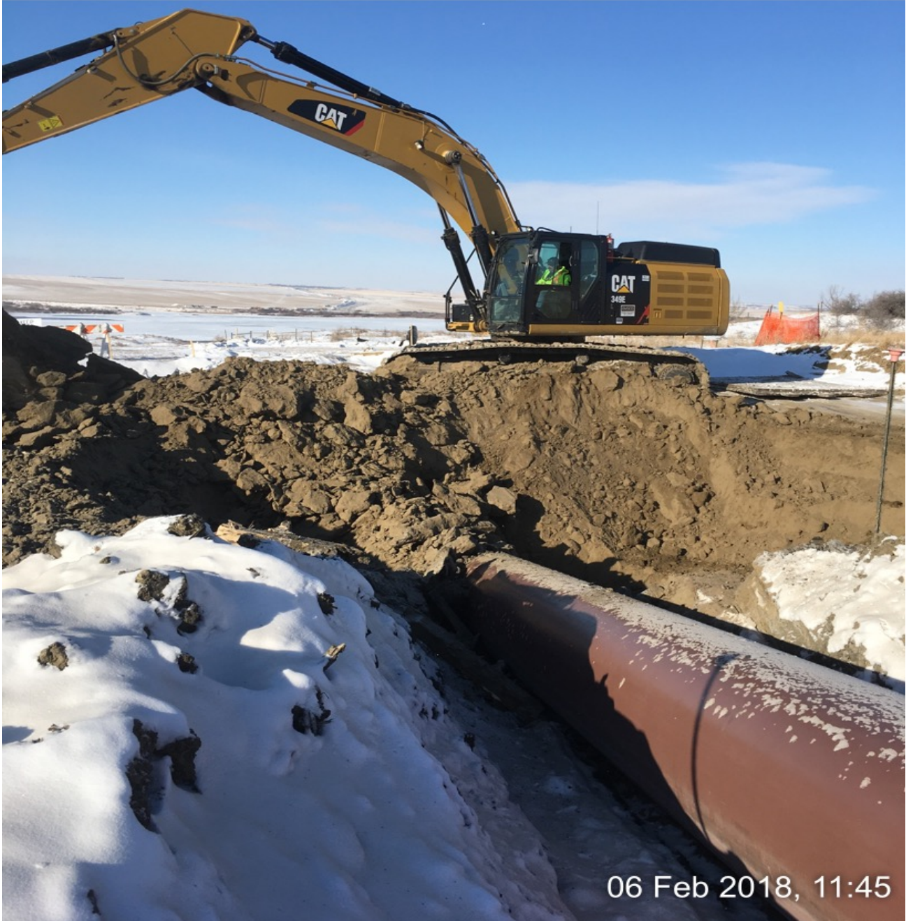
BACKFILLING DITCH LINE
