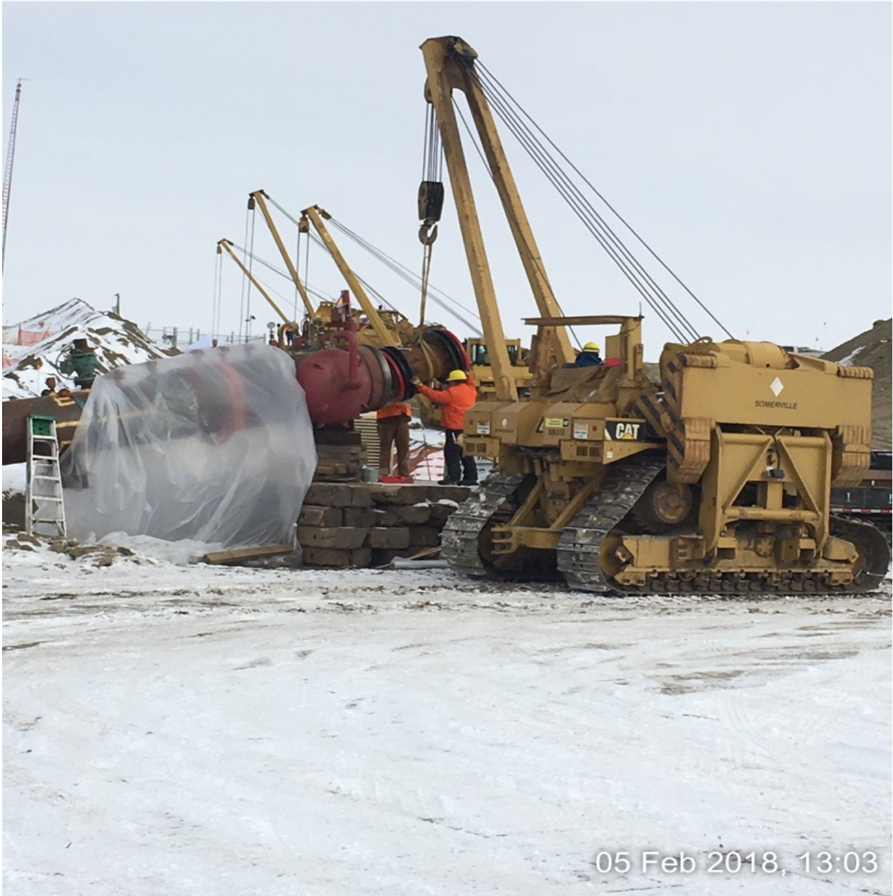
INSTALLING PIGS AT TEST HEAD
