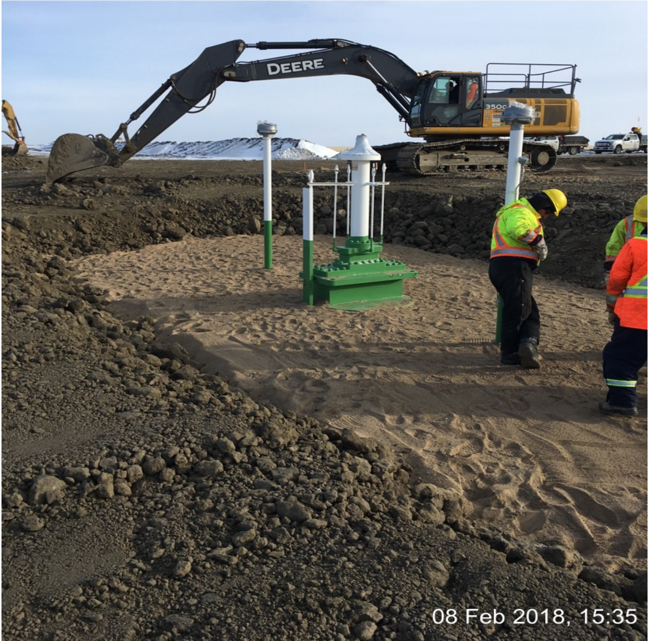
BACKFILLING VALVE NUMBER SEVEN
