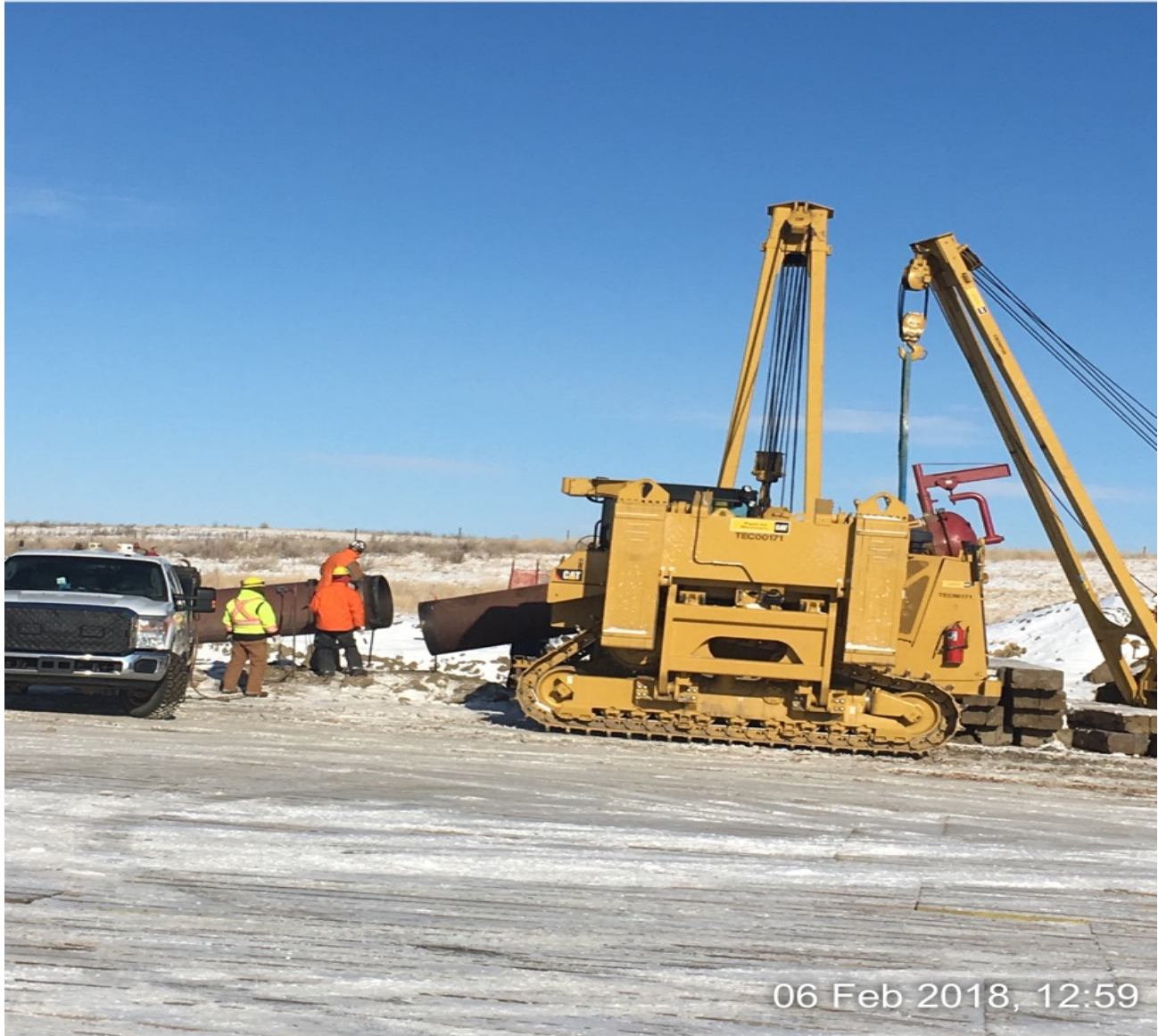
CUTTING TEST HEAD OFF AT EXIT POINT
