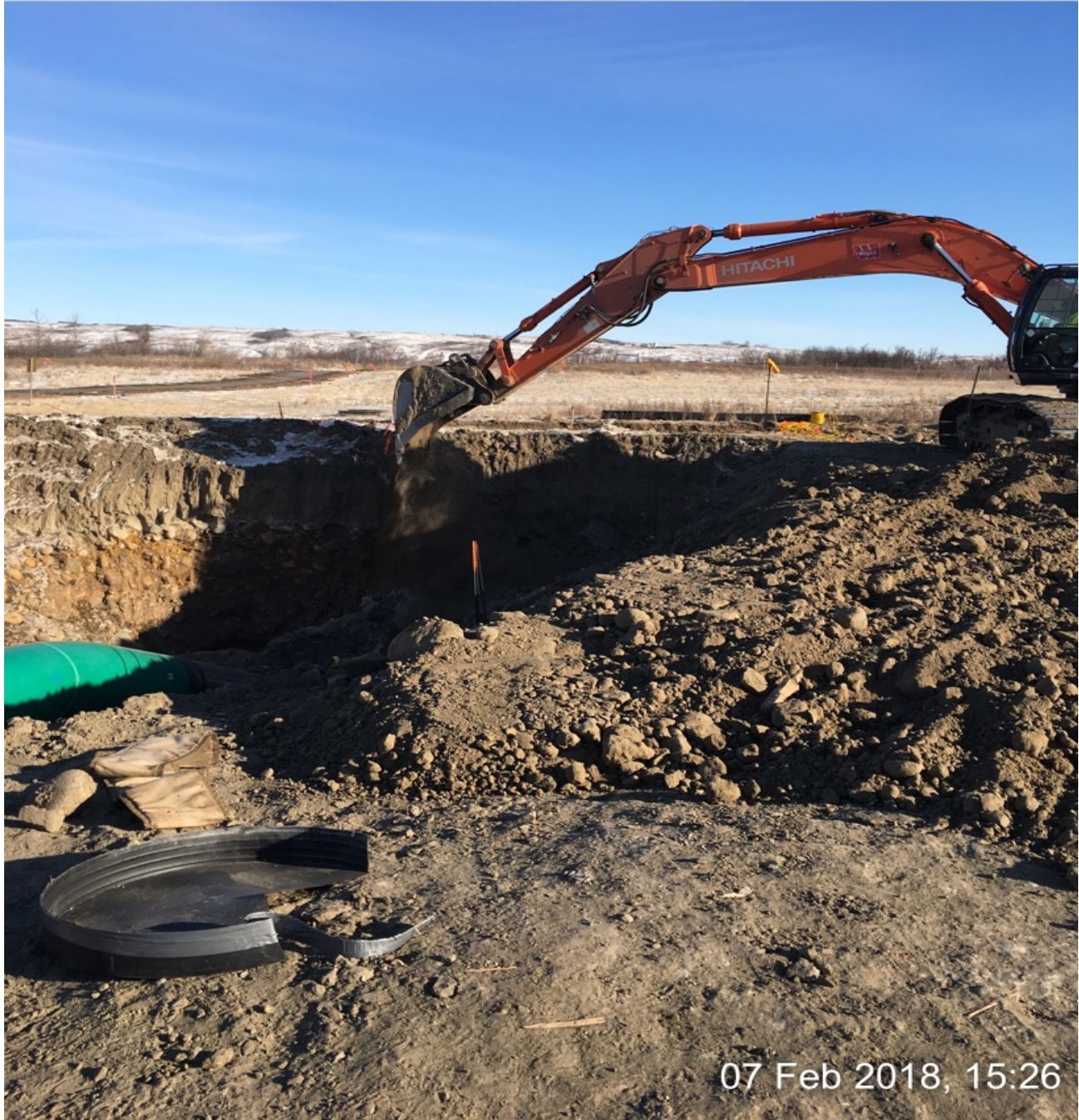
BACKFILLING ENTRY POINT
